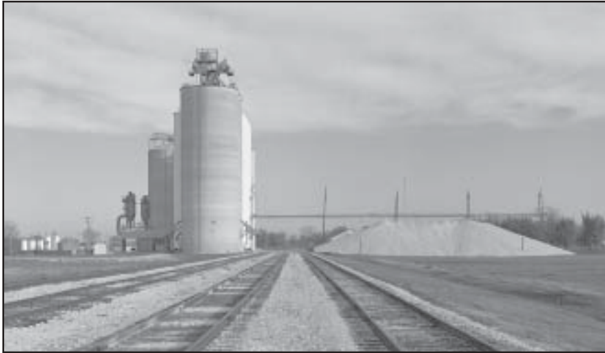
Pro Cooperative grain elevators, 1994.
