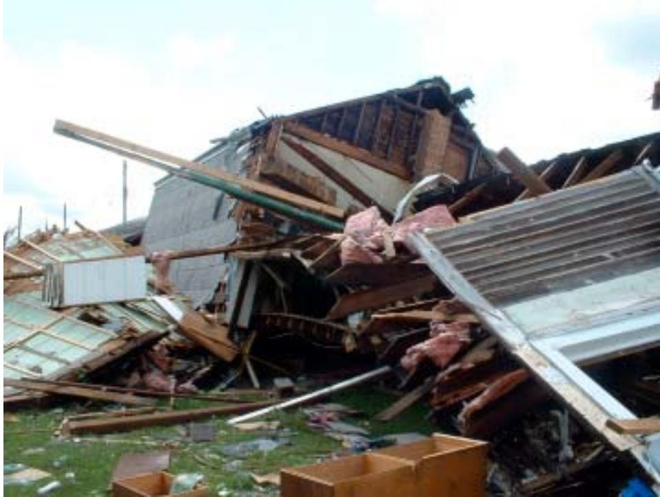
Looking south at home on the north side of town. Home destroyed with roof gone. Home was “twisted off” foundation resulting in failure (F2).
