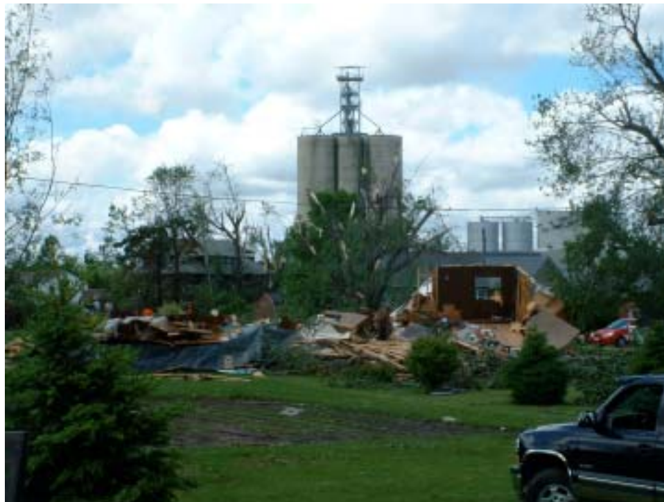
Looking south from northeast corner of town. Home which suffered complete failure. Note lack of major damage next to home which resulted in F2 rating (F2).
