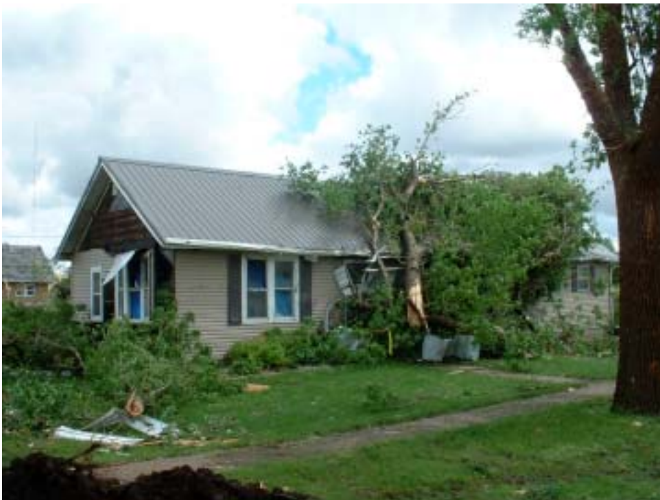
Looking northeast on northeast side of town. Home with tree down on it (F0).
