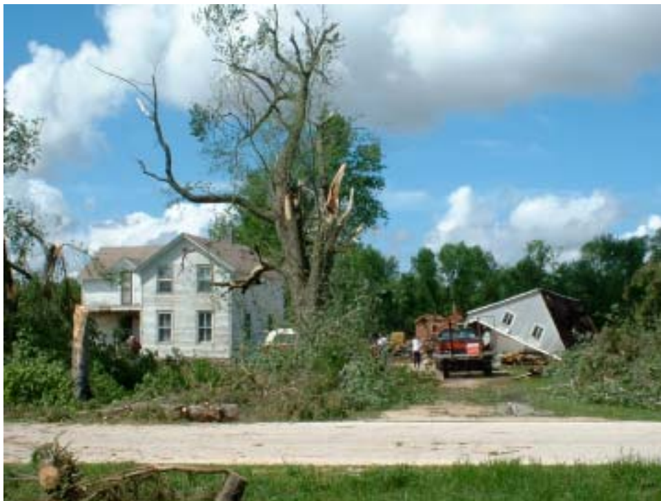
Looking south at home on the north side of town. Home destroyed with roof gone. Home was “twisted off” foundation resulting in failure (F2).
