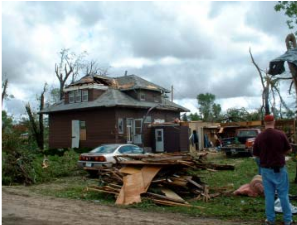
Looking east from east side of town. Home with garage destroyed but main home with minor damage (F1).
